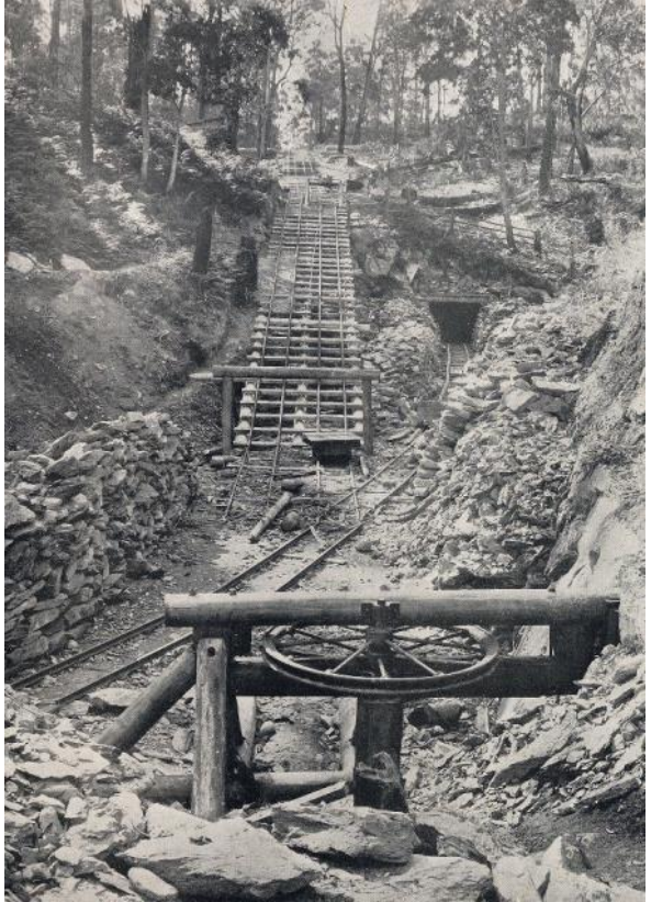
Tasmanian Shale Oil Co haulage and adit 1911.
