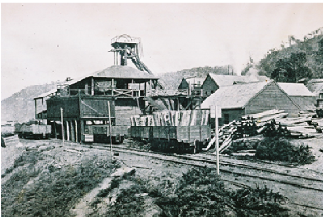
Above - Mine props and coal loading facilities at Lithgow.
