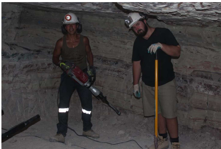
Photo 5. Adam Abersteiner and Logan Williams deepening the Adit face floor with a brand new Chinese Dragon electric hammer designed to break 20 cms of concrete. The floor is a half metre thick of tough silicified sedimentary injectite and given Logans size and posture we had to buy a special tool to drop the floor for the taller workers.
