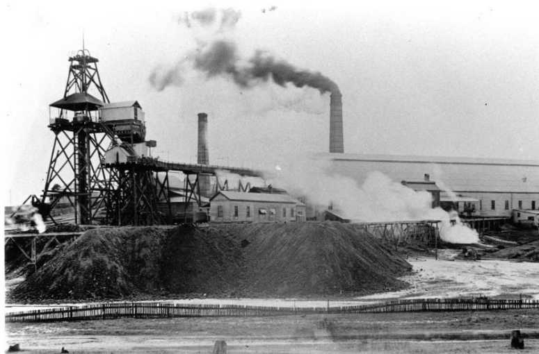
Figure 3. Headframe, (No.1), battery and retort house of Scottish Gympie Gold Mining Company, c 1900.
